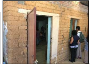
Cracks from earthquakes
