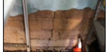
Cracks from earthquakes
